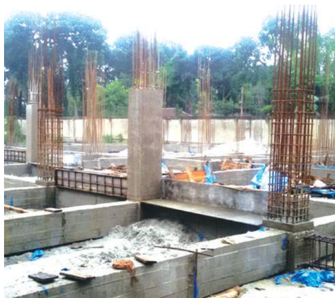
Construction of CRP-Manikganj starts
