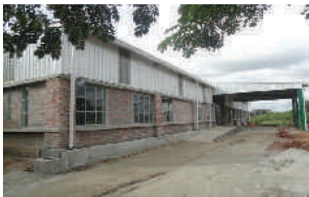
Newly constructed workshop for production of wheeled mobility aids and assistive devices at CRP-Ganakbari
