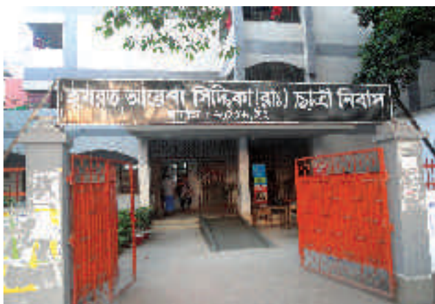
Made accessible for wheelchair user by CRP
