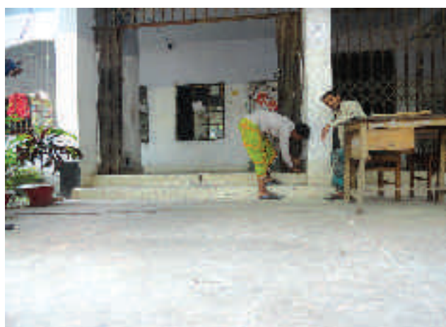
Inaccessible hostel for wheelchair user
