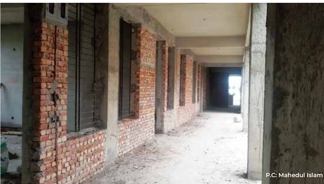
CRP-Manikganj Vocational Training and Rehabilitation Centre construction ongoing
